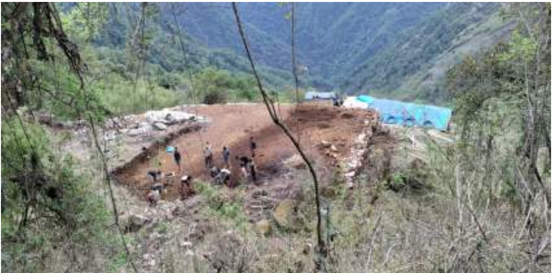
Construction of Survey Camp
