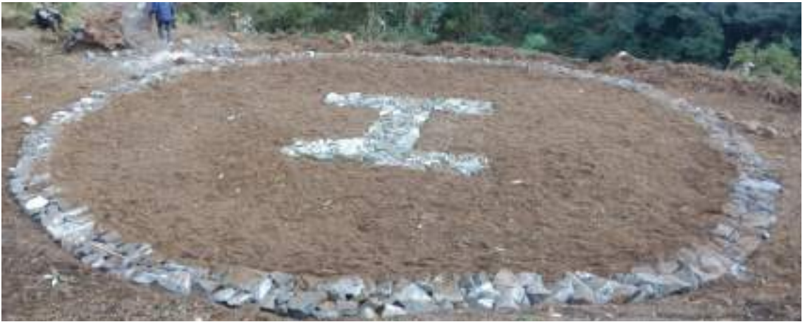
Constructed Helipad in Project Site
